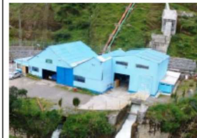
CH Baños IV = 5.0 MW
