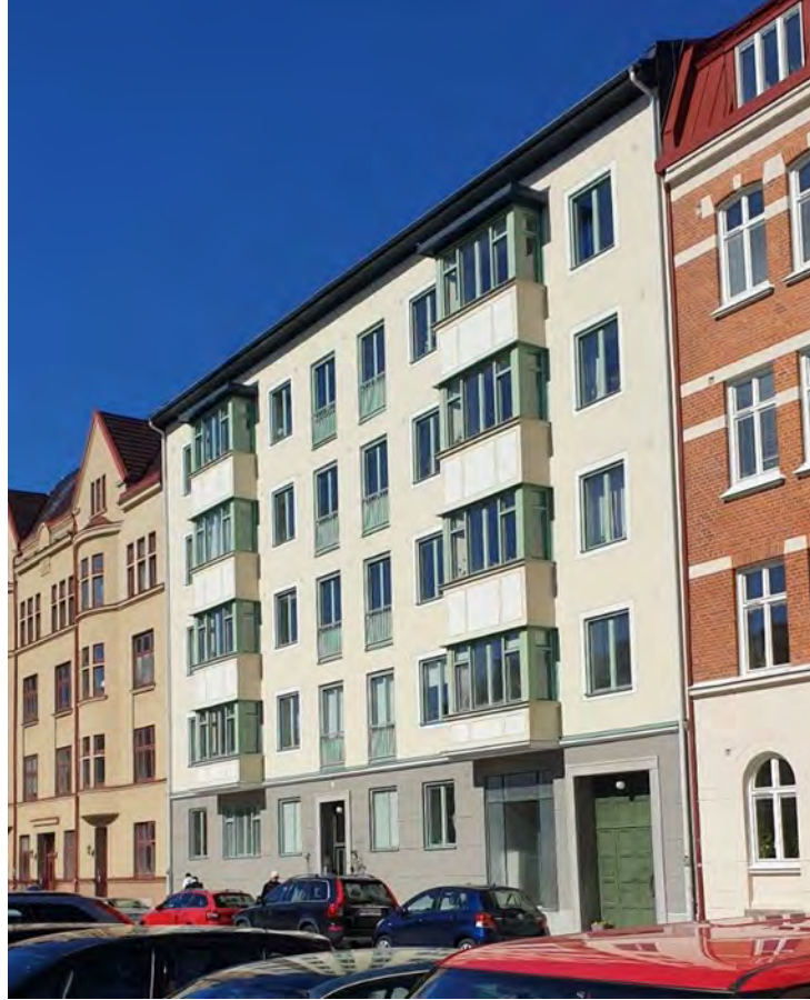
Fig. 17. Photo of Building 1 which is a 6-story residential building containing multiple apartments located in central Malmö, Sweden. Photo: Erik Kimblad.
