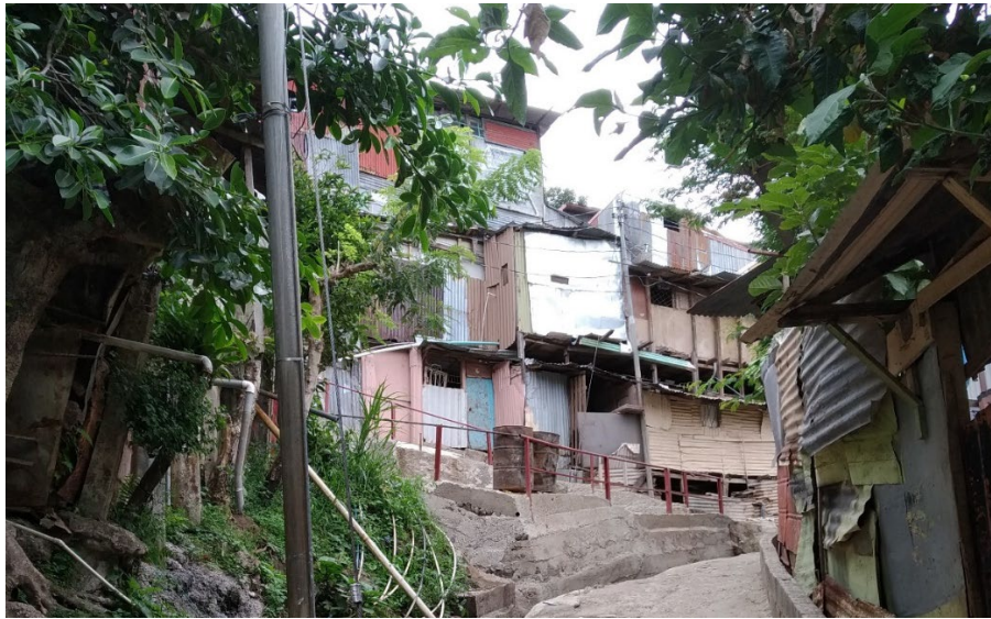
Figure 1. Multistorey buildings in La Carpio (Author's photo)
