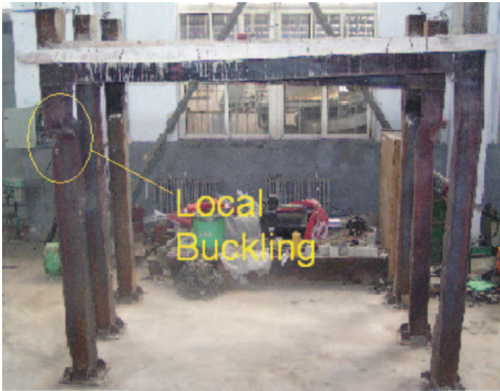
Figure 12. Photograph of the frame at the conclusion of the furnace test showing the formation of local buckling on column 1 close to the connection. (The color version of this figure is available online.)
