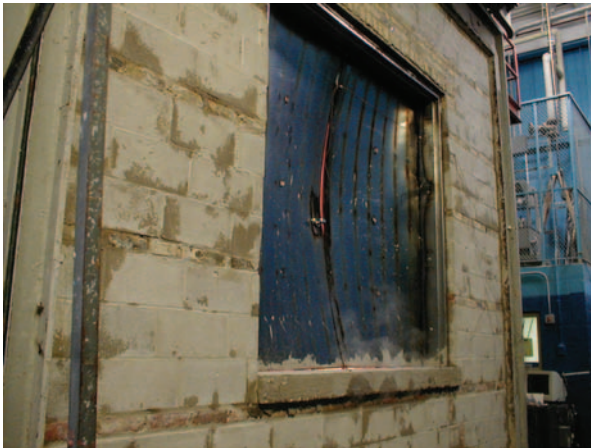
Figure 12. Photograph of fire door assembly during the test after 1 hour (The color version of this figure is available online).
