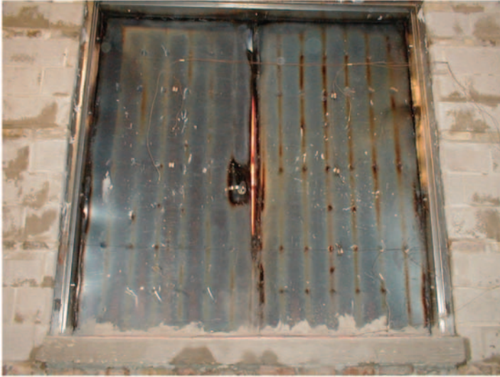
Figure 10. Photographs of the fire doors during the fire endurance test after 1 hour (The color version of this figure is available online).
