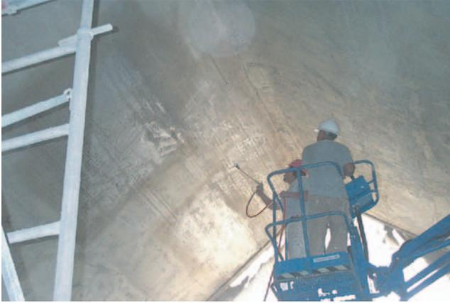
**Figure 8.** Overhead application of fire insulation over an FRP-strengthened concrete roof slab in a manufacturing plant (photo courtesy Fyfe Co. LLC, San Diego). (The color version of this figure is available on-line.)
