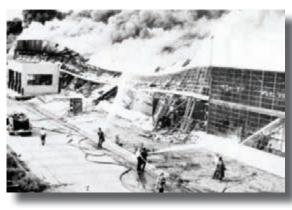
At one time, roof assemblies were assumed to be fire safe if the deck and its supports were of metal, particularly when the fire hazard of the building's contents were considered low to moderate. This type of roof construction was classed as "non-combustible" even though the vapor barrier, adhesive and roofing used were combustible.
