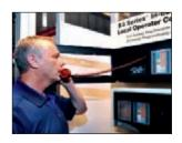
notification requirements of LOCs as mandated by the U.S. Department of Defense in its Unified Facilities Criteria (UFC) document 4-021-1. A telephone and 16 programmable switches allow this LOC-TEL to direct pre-recorded and live voice messages to any designated area within a facility.
