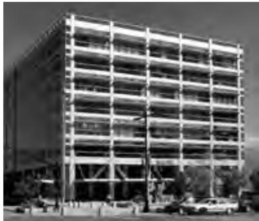
GSA renovated the Wallace F. Bennett Federal Building in Salt Lake City in 2001, upgrading the seismic design features to ensure a safe, durable workplace. Correcting performance problems of some mid-century buildings can be a challenge. In this case, an energy-efficient curtain wall system was added to allow more natural light to enter the building.
