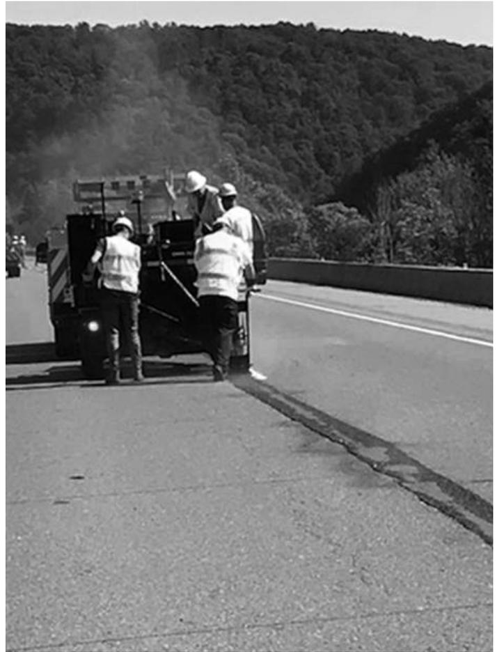
aggregate topping stone to be applied to the surface of the mastic. This fine stone improves the surface friction properties of the repair without additional costs to the roadway owner.
