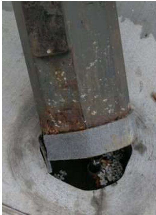
Photo 1: Traffic Pole at the point of encasement.
