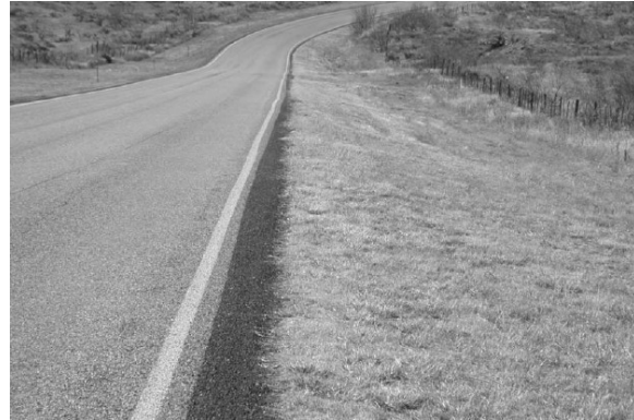
Fog seal applied along the edge of pavement (from TxDOT Project 0-4396).
