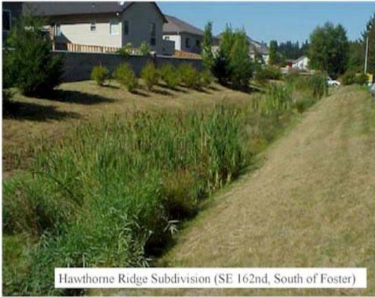
A Vegetated Swale is a broad, shallow, trapezoidal or parabolic channel, densely planted with a variety of trees, shrubs, and/or grasses. It is designed to attenuate and in some cases infiltrate runoff volume from adjacent impervious surfaces, allowing some pollutants to settle out in the process. In steeper slope situations, check dams may be used to further enhance attenuation and infiltration opportunities.
