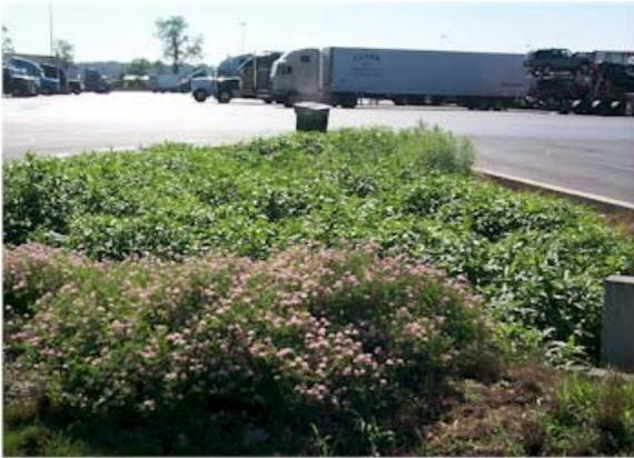
Filters are structures or excavated areas containing a layer of sand, compost, organic material, peat, or other filter media that reduce pollutant levels in stormwater runoff by filtering sediments, metals, hydrocarbons, and other pollutants.
