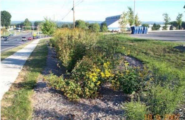
Subsurface Infiltration Beds provide temporary storage and infiltration of stormwater runoff by placing storage media of varying types beneath the proposed surface grade. Vegetation will help to increase the amount of evapotranspiration taking place.
