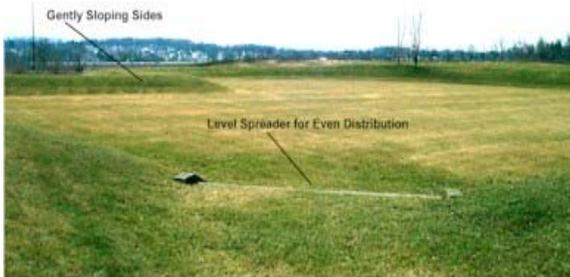
An Infiltration Basin is a shallow impoundment that stores and infiltrates runoff over a level, uncompacted, (preferably undisturbed area) with relatively permeable soils.
