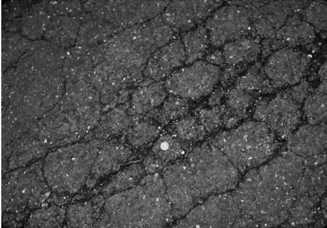
*This picture illustrates moderately severe fatigue cracking. The cracks have formed a pattern, and are slightly spalled. However, there is no sign of pumping.*
