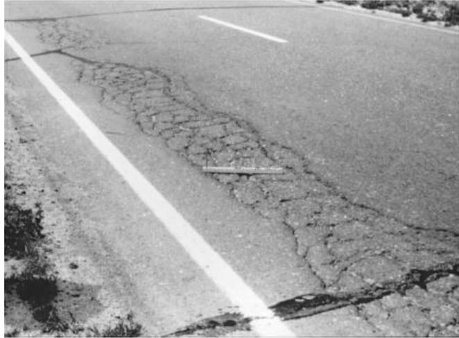
*This is an example of high severity fatigue cracking. The pattern is well-developed, and the interconnecting cracks are spalled. The cracks are deep, and some of the sections are loose enough to move with passing traffic.*
