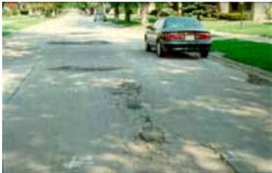
*Before paving, a roadway must be prepared through proper pothole repairs, base repair, crack sealing, or scratch and leveling courses to address surface irregularities and provide a uniform foundation.*
