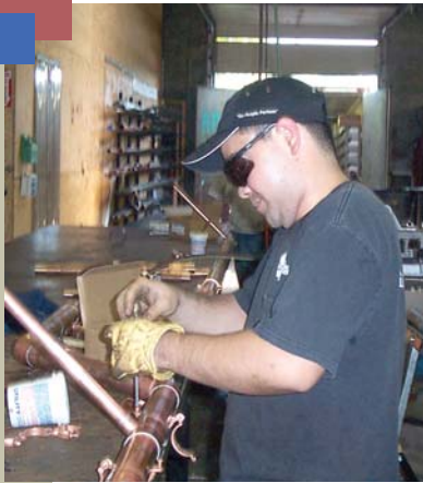
A journeyman prepares to solder fittings in a piping assembly.
