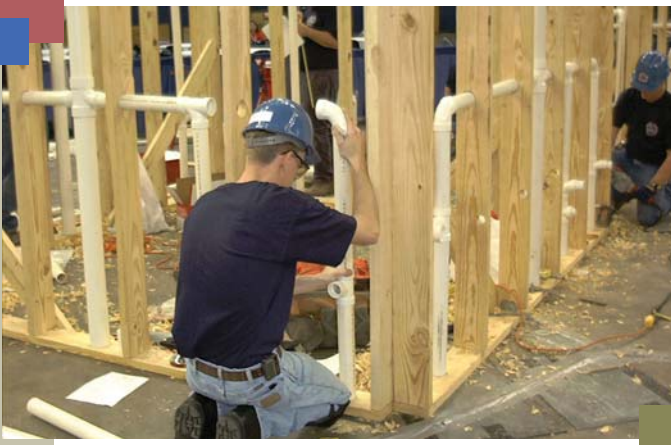
Apprentices assemble PVC piping in a training exercise.
