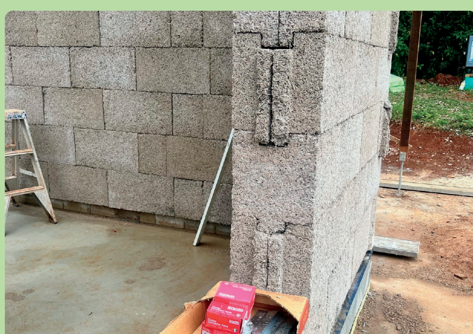
Hempcrete blocks homes (in Australia)
