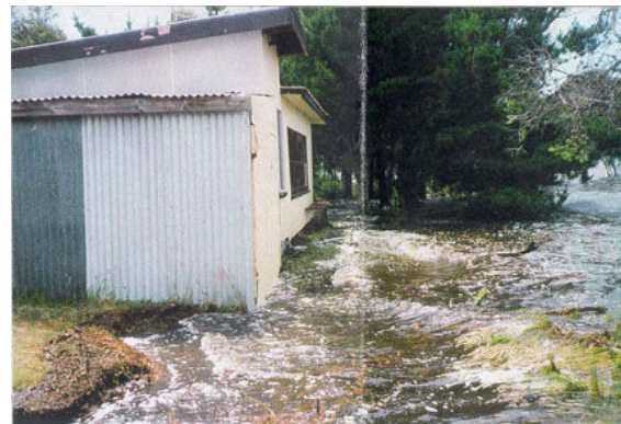
Figure 5: A storm surge at Anson’s Bay during 1993. Several floods of this magnitude or greater have occurred during the last few decades, impacting on shacks built on the former crown coastal reserve strip. However freehold blocks to landwards have had little or no flood impact, implying that the crown reserve would have provided adequate flood buffering for residences if it had been permitted to perform this function. Photo: Richard Mason, Break O’Day council.
