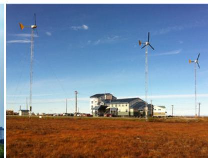
Three 10-kW wind turbines provide behind-the-meter energy for a school in Alaska. *Photo credit: Bergey WindPower*
