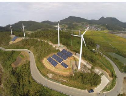
Four 100-kW wind turbines are part of the isolated grid on Gasado island, South Korea. *Photo credit: Korea Electric Power Corporation*
