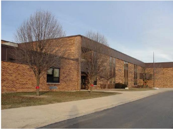
15711 Bell Road Homer Glen, Illinois 60491 Original Year built: 1981 Additions built: 2004 Size: (2) Stories, 101,710 g.s.f. (est.)
