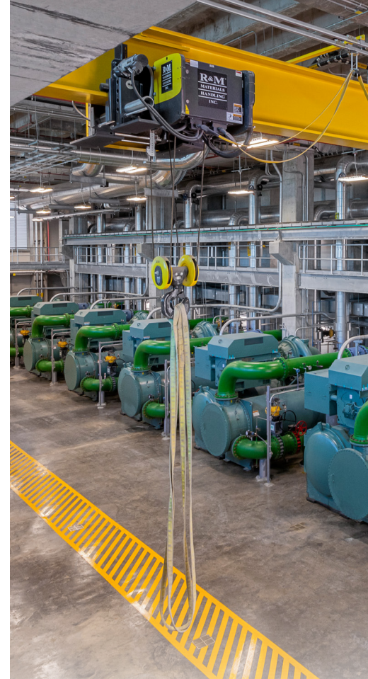
Six new 2,500 ton chillers in the chilling station supporting the Dell Medical School and main campus.
