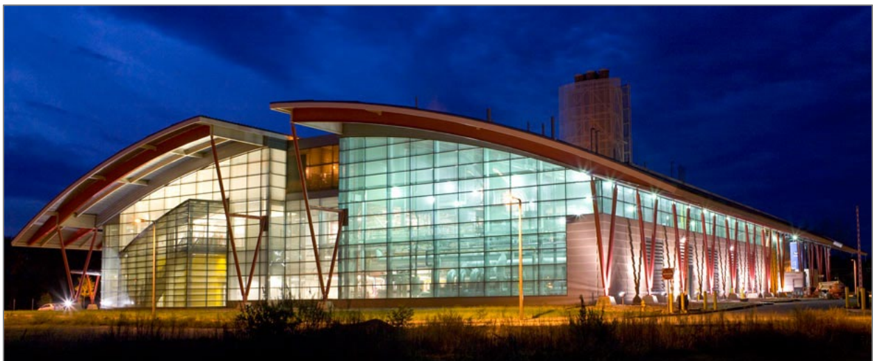
Figure 4. UMass Amherst Central Heating Plant
