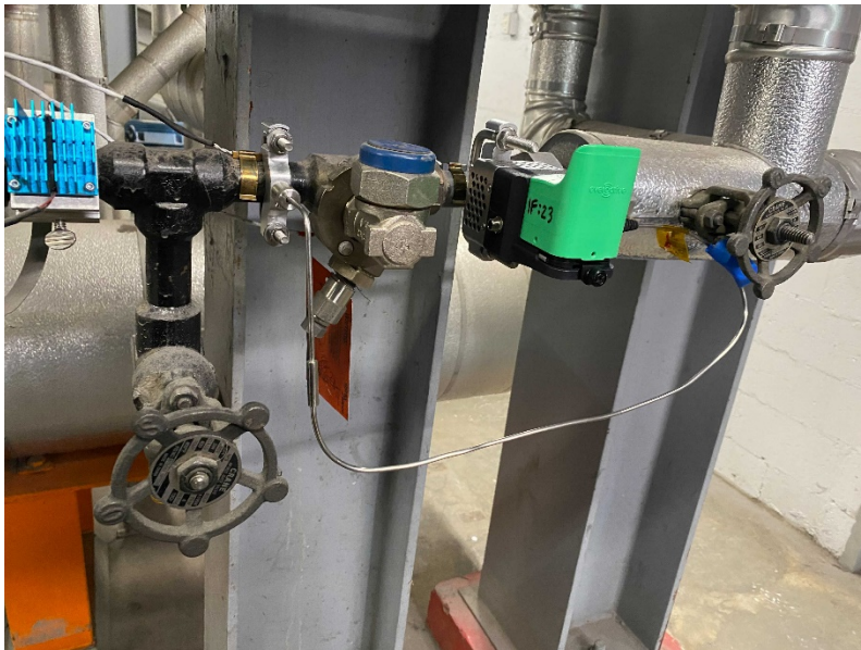
Figure 3: STM installed in at an UVA steam trap.
