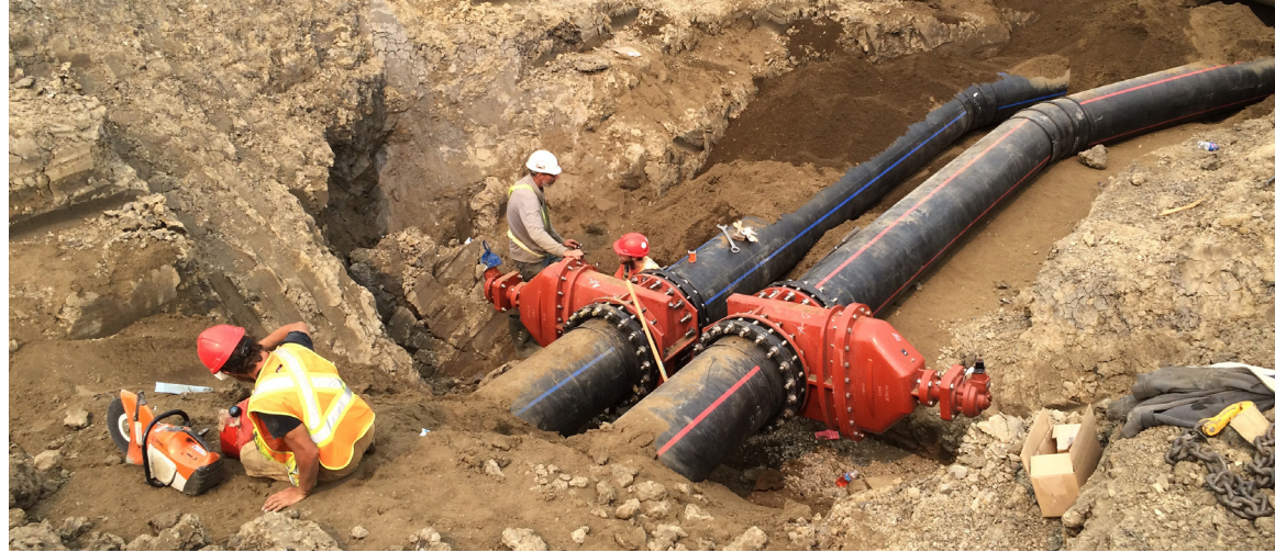
Photo: Installation of stage one distribution pipes
