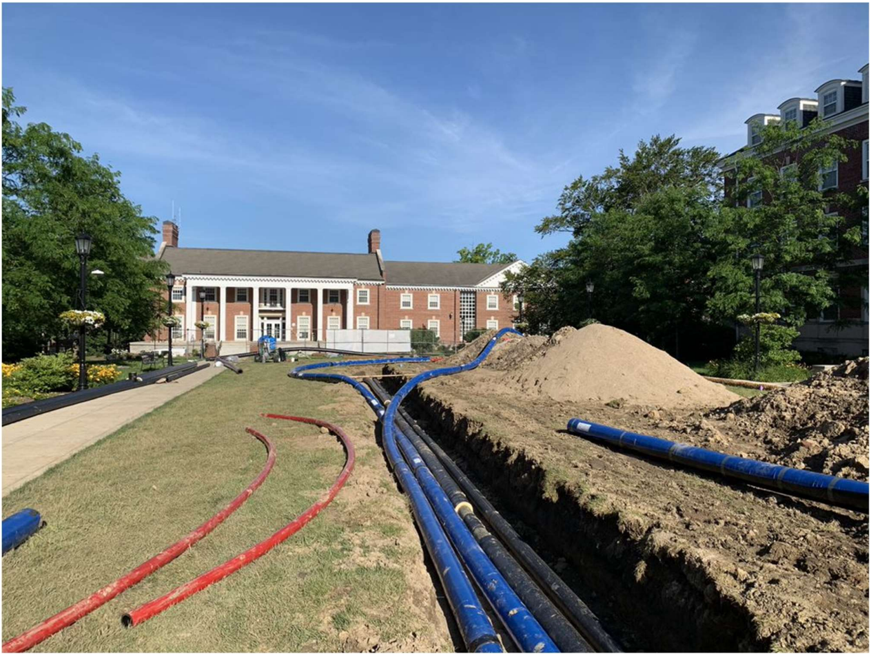
Flexible piping laid into a trench
