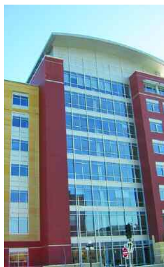
Elmer L. Andersen Building
