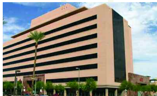
411 Building - Arizona State University
