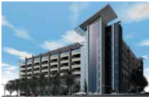
Omaha Park VIII & Tunnel
