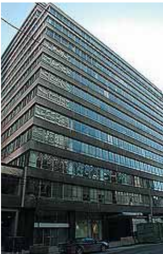
Richmond-Adelaide Centre - 111 Richmond St. W.
