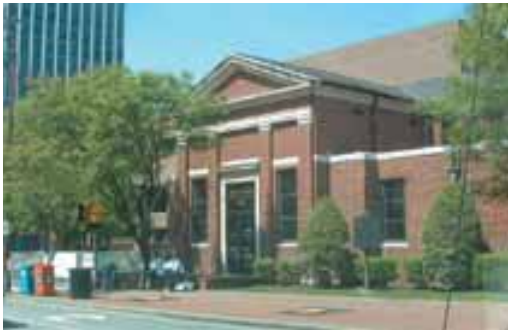
Ben West Building
