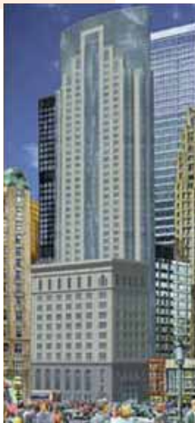
One King West Condominium
