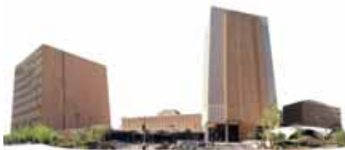
Maricopa County West Courts Complex
