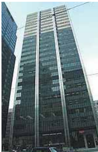
Richmond-Adelaide Centre - 120 Adelaide St. W.
