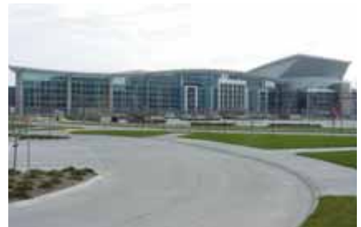
Qwest Convention Center/Arena Omaha
