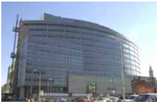
City and County of Denver Office Building
