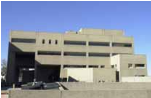
Police Detention Facility
