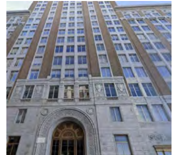
Vicinity Energy - 320 S Boston
