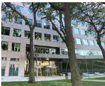
Vicinity Energy - 500 Tech
