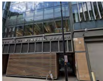
Vicinity Energy - 650 Kendall
