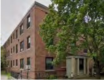
Vicinity Energy - 700 Main St
