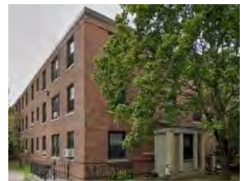
Vicinity Energy - 700 Main St
