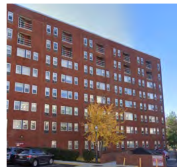
Vicinity Energy - East Front
