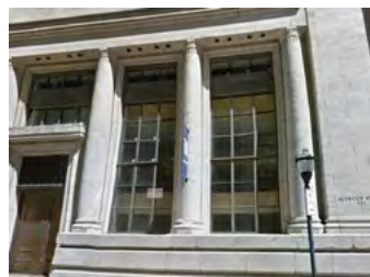
Vicinity Energy - East Redwood
