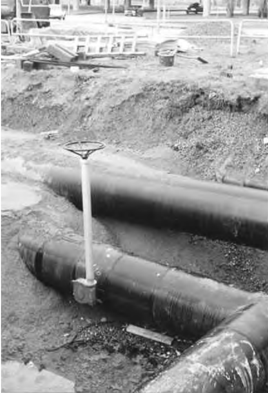
Figure 6-9. Direct-buried valve with mechanical actuation.
