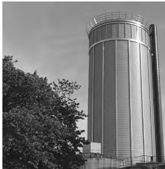
Figure 6-6. Thermal storage tank used for maintaining static pressure in system.
