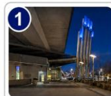
False Creek Energy Centre
