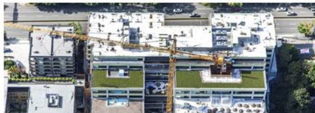
1101 Dexter Installation with Firestone 30 year TPO and Firestone SkyScope Garden Roof. Contractor - Cobra BEC.
