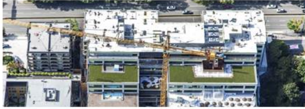
1101 Dexter installation with Firestone 30 year TPO and Firestone SkyScope Garden Roof. Contractor - Cobra BEC.
