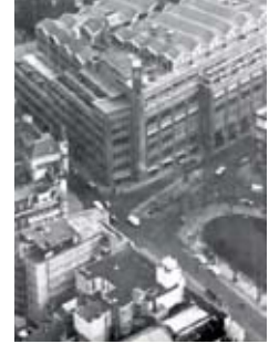
Figure 11.5: The 1930s building on Rembrandtplein Amsterdamsche Bank's old head office was drastically renovated and extended by Amro Bank in 1966-1972. In April 2002 the bank left the building. Source: ABN AMRO online archive
