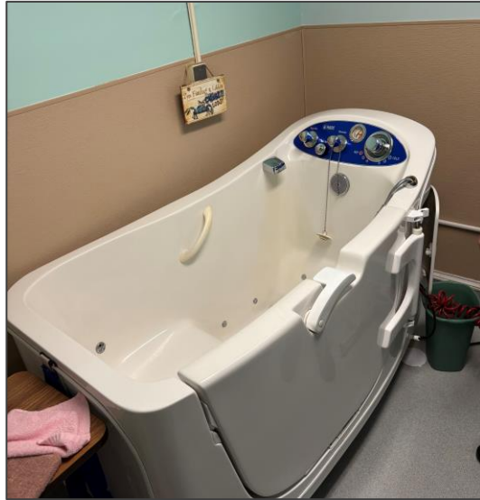
Whirlpool tub (w/ staining)
