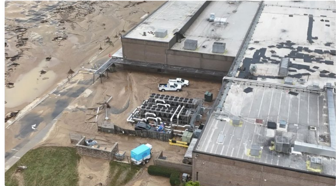
Baxter's North Cove manufacturing facility after Hurricane Helene in Marion, N.C., on Oct. 2, 2024. Retrieved from Aerial Lens on October 04, 2024
