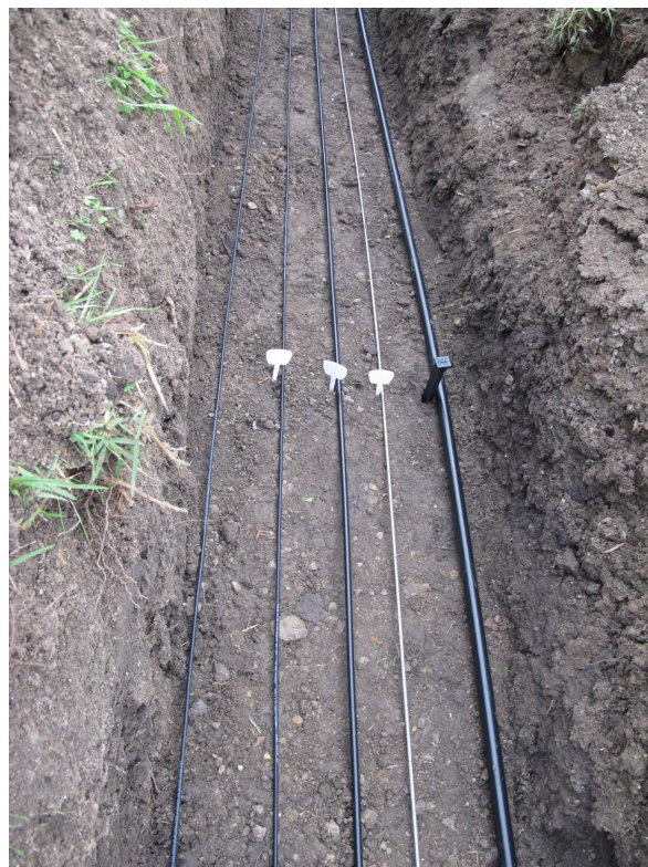
Fiber-optic cables after being installed in a trench. Image Credit: J. Ajo-Franklin
