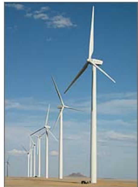
These wind turbines near Lamar, Colorado, are part of the 162-MW Colorado Green Wind Farm. Each turbine produces 1.5 megawatts of electricity.
