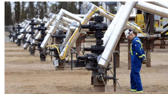
A Statoil field worker looks at oil well heads on a well pad at the company's oil sands operation near Conklin, Alta
