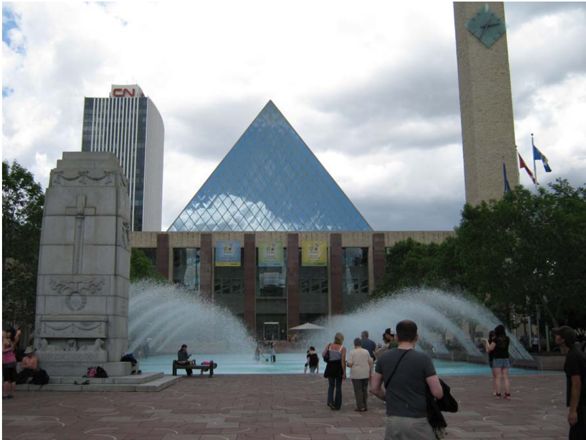
Photo 2: Edmonton City Council Chambers
