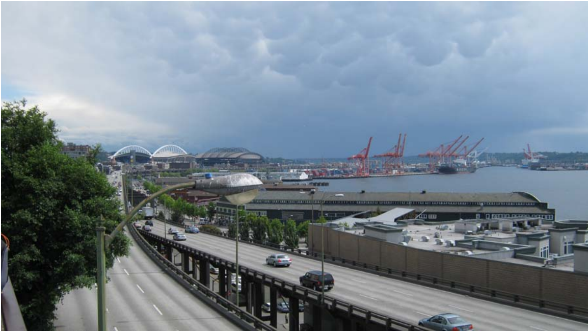
Photo 17: Motorway is being removed
