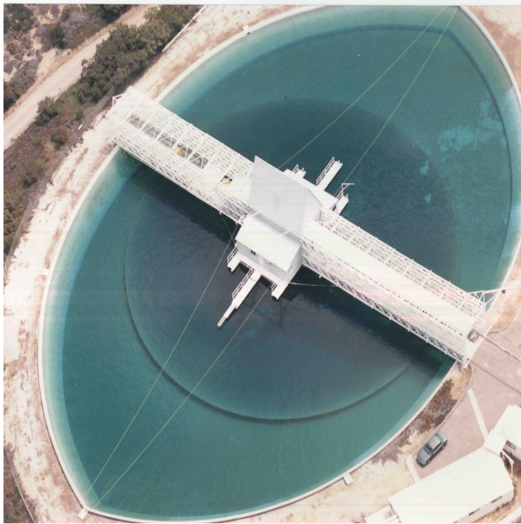
Drawing 2: Aerial photo of facility. The bridge structure has no piers or supports in the pond.
