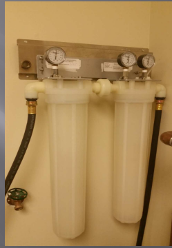
5 micron filter 0.1 micron bacterial filter
